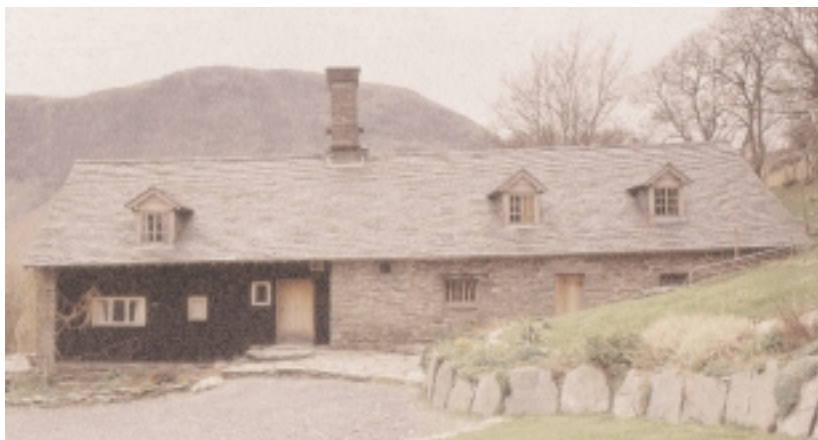
The once dilapidated farmhouse of Nannerth Ganol, Rhayader, has been restored to become a habitable building again.
